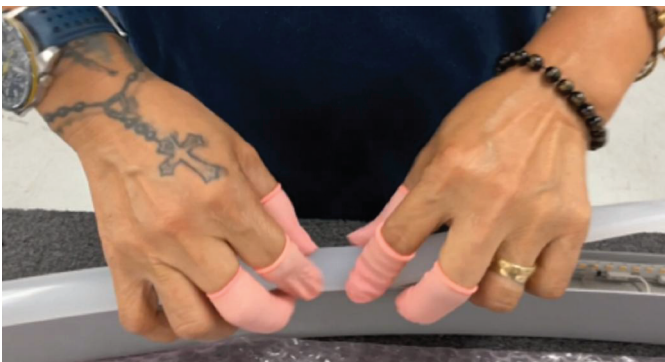
Insert the diffuser in place
