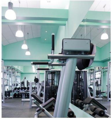
The industrial-style dome is a workhorse equipped with a clear prismatic diffuser that maximizes the pendant's efficacy, delivering high light outputs suitable for the high ceilings of warehouses and superstores. An optional White refractor is available.
